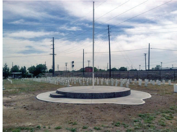
Flag pole area after construction.
